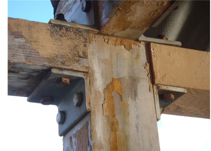
post-to-post beam bracket
